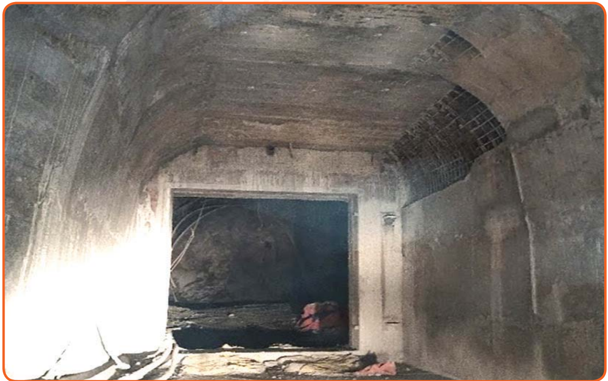
MISTRI KHOLA HEP BULKHEAD GATE
