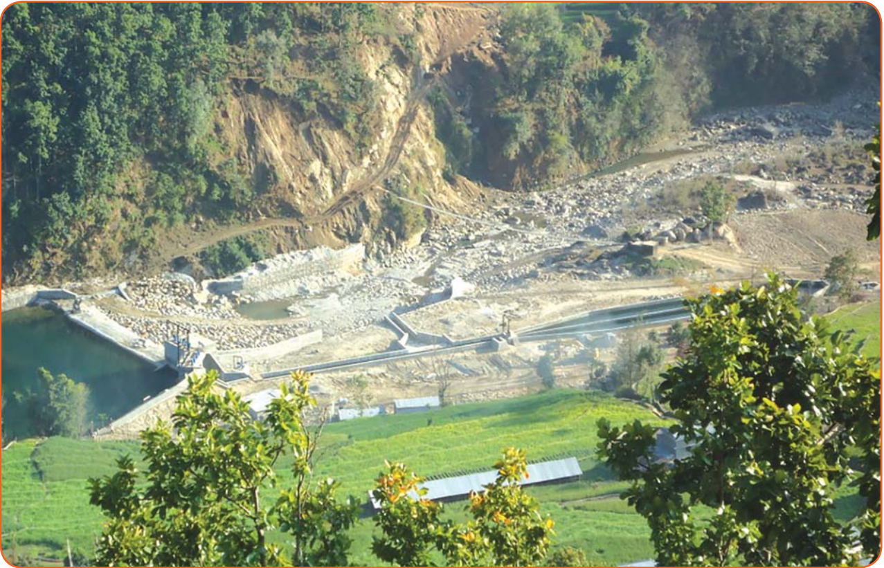
TADI KHOLA HEP HEADWORKS
