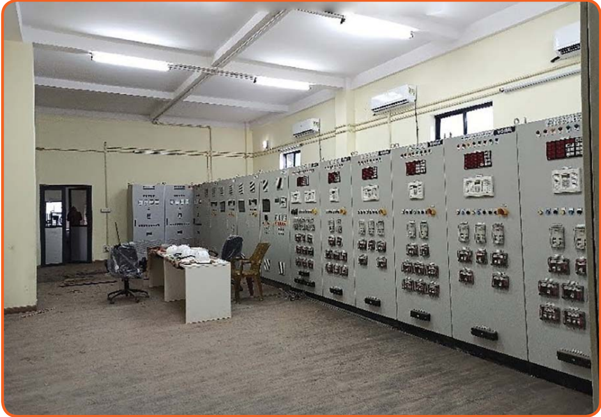
MISTRI KHOLA HEP CONTROL ROOM
