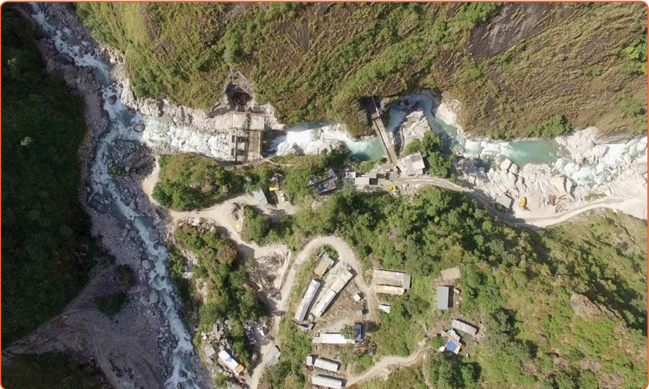
MISTRI KHOLA HEP HEADWORKS AERIAL VIEW
