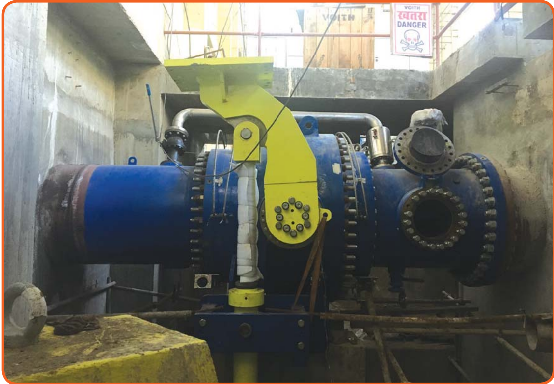
MISTRI KHOLA HEP- MAIN INLET VALVE AT POWERHOUSE
