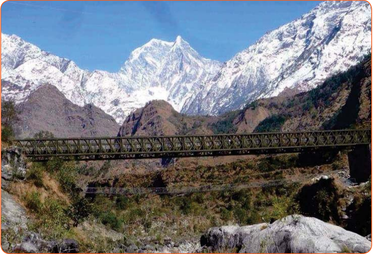
MISTRI KHOLA HEP BAILEY BRIDGE OVER KALIGANDAKI RIVER INSTALLED BY MOUNTAIN ENERGY NEPAL LTD.
