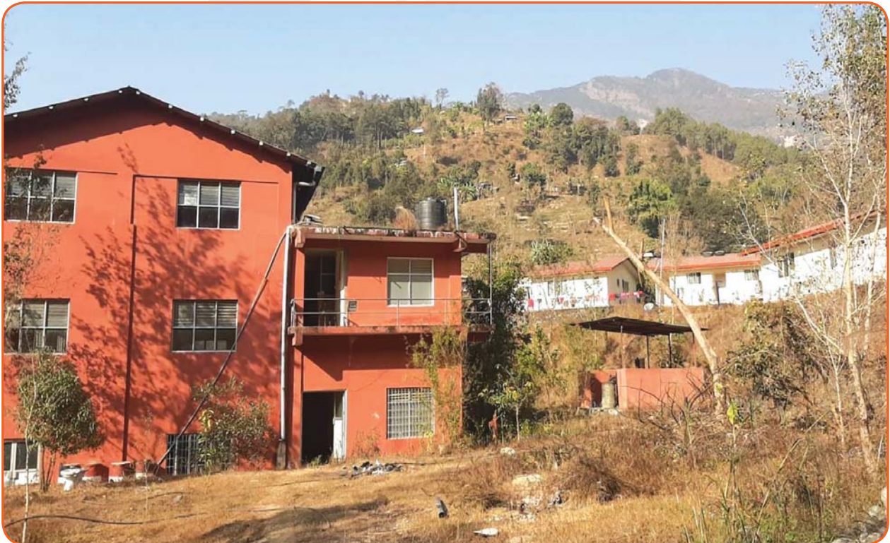
TADI KHOLA HEP POWERHOUSE AND EMPLOYER'S CAMP
