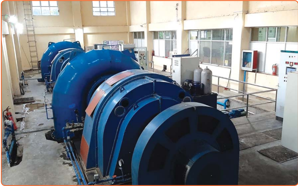
TADI KHOLA HEP -TURBINE & GENERATOR
