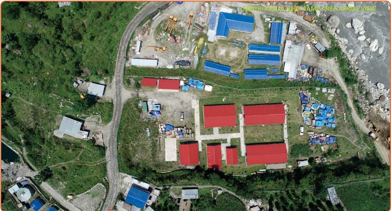
MISTRI KHOLA HEP CAMP AREA AERIAL VIEW
