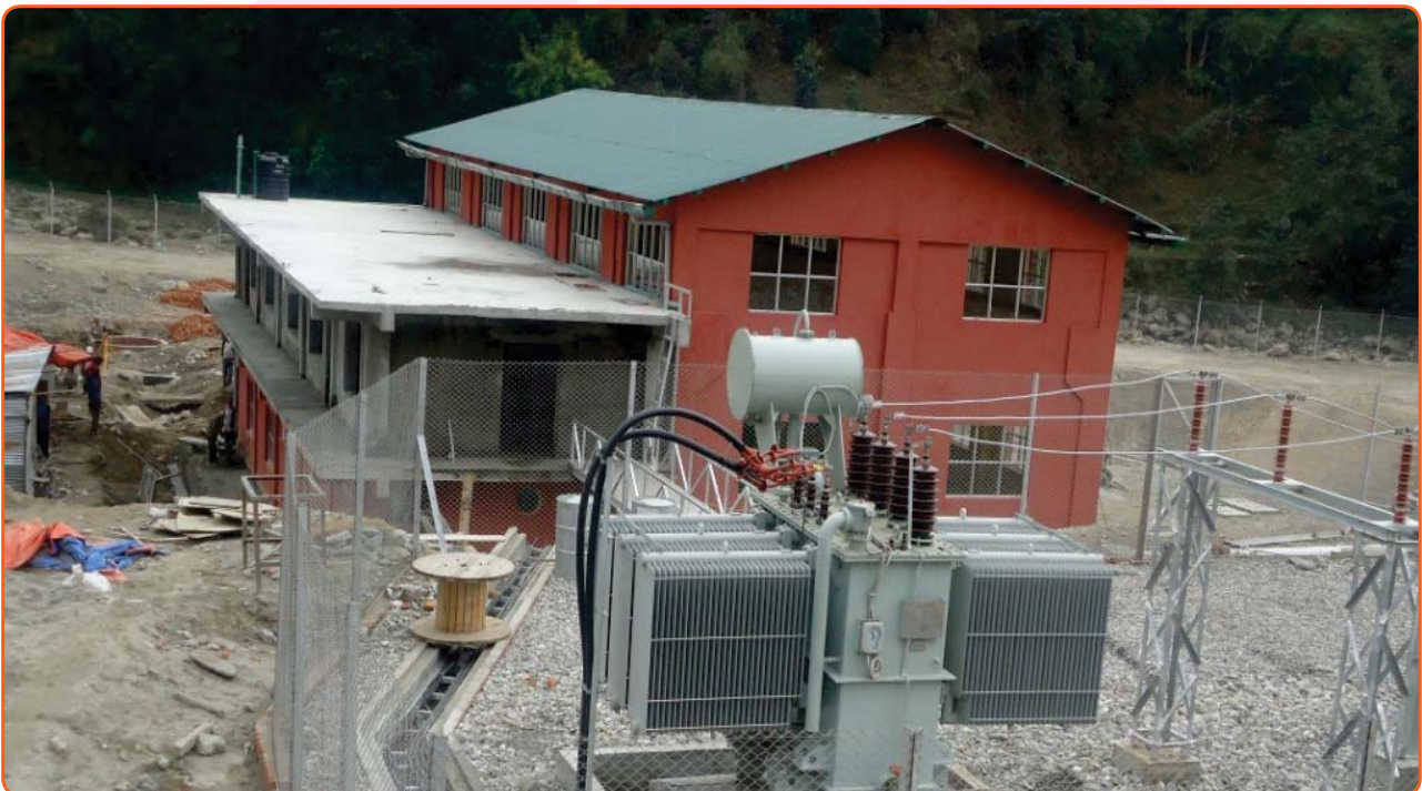
TADI KHOLA HEP POWERHOUSE
