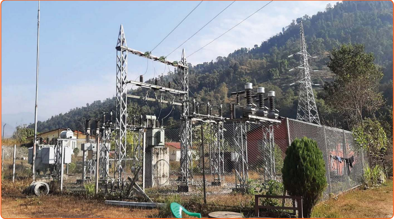
TADI KHOLA HEP SWITCHYARD
