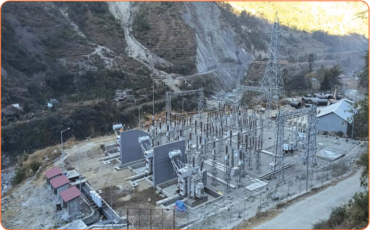
MISTRI KHOLA HEP SWITCHYARD
