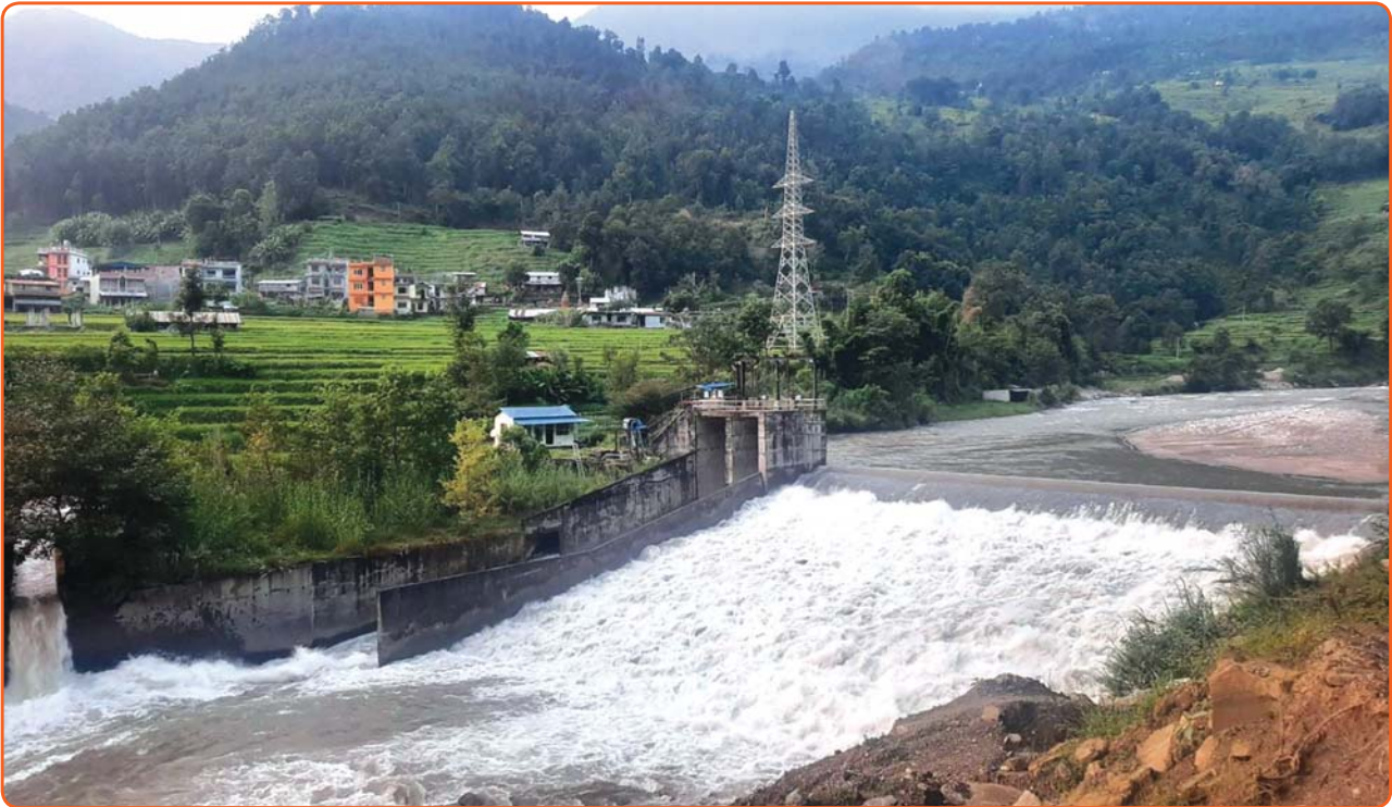
TADI KHOLA HEP-HEADWORKS
